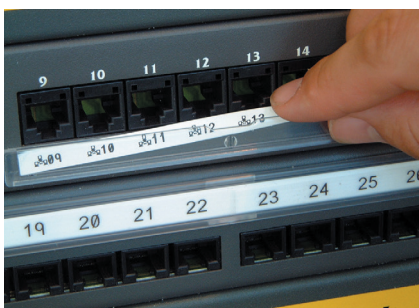
Punch block & patch panel labels
